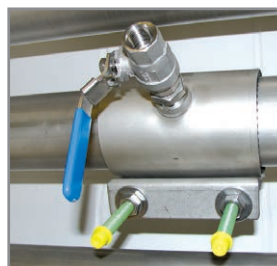
B Spot drilling collars
